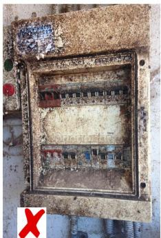
Must be maintained and protected to prevent electric shock or fire
